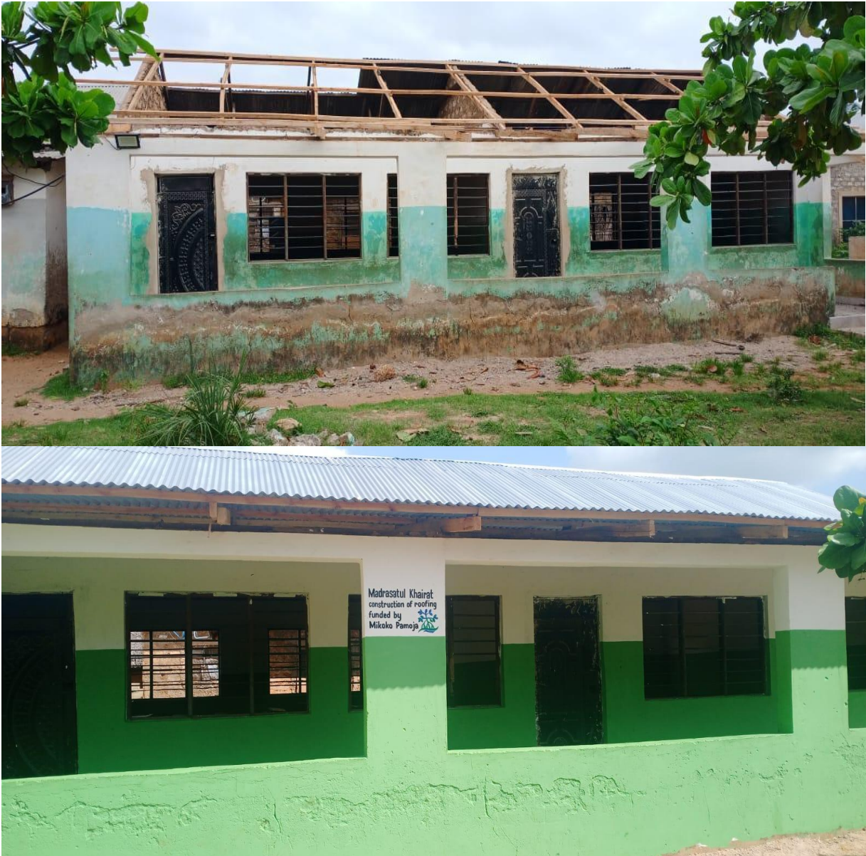
Figure 13. The renovation of the madrasa roofing has been completed, addressing structural needs to enhance the learning environment.
