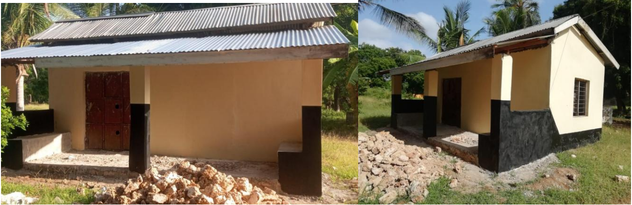
Figure 14. The water project continuation from 2023 is progressing steadily (top) and the proposed endowment ( Waqf ) project in Makongeni to provide accommodation for madrasa teachers (below)
