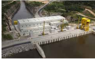
Côte d'Ivoire Soubré Hydroelectric Verified to Verra VCS by 4K Earth Science Private Limited
